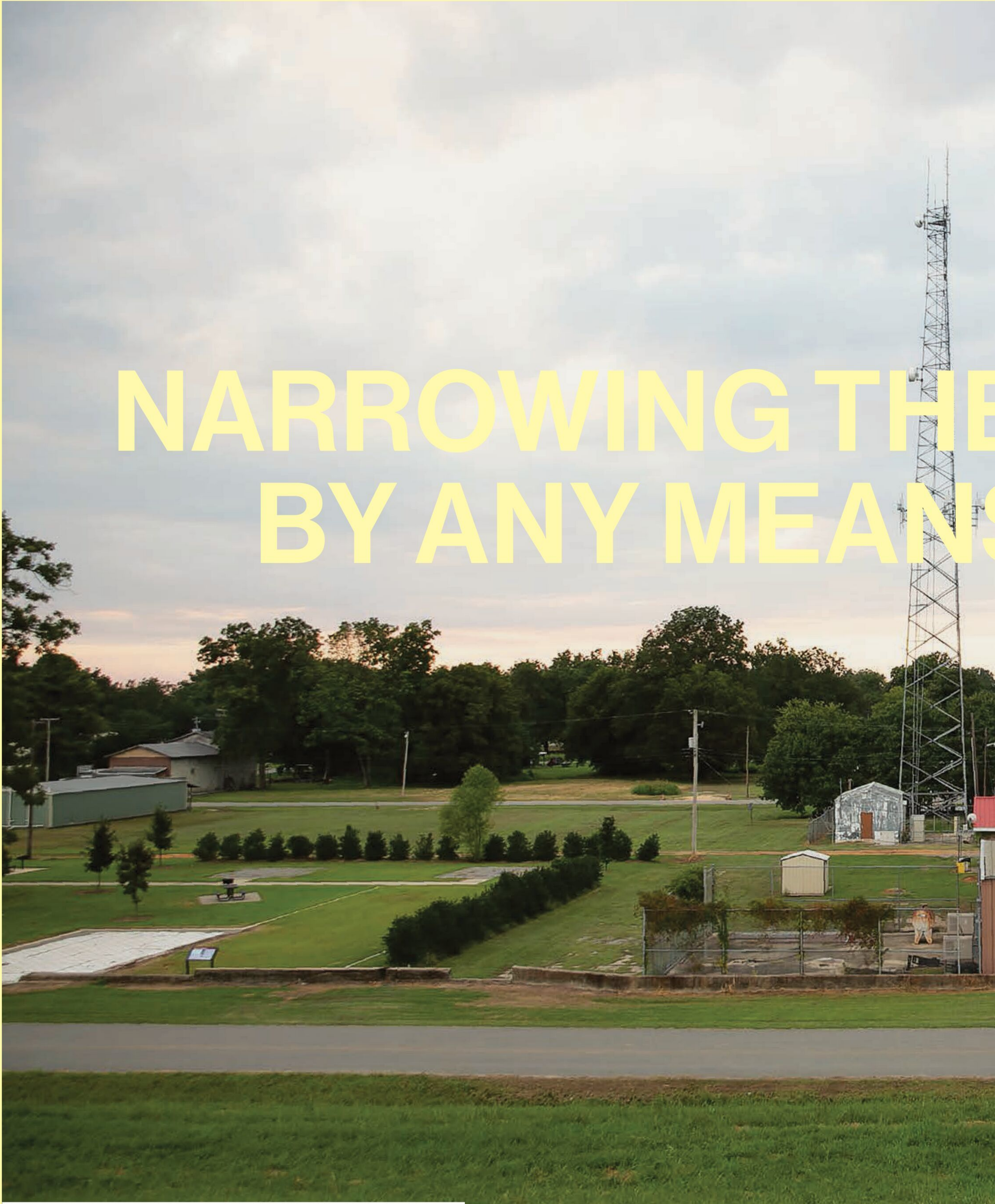
▲ A 180-FOOT RADIO TOWER IN ARKANSAS CITY, ARK., IS PART OF A PLAN TO FILL GAPS IN U.S. BROADBAND COVERAGE
