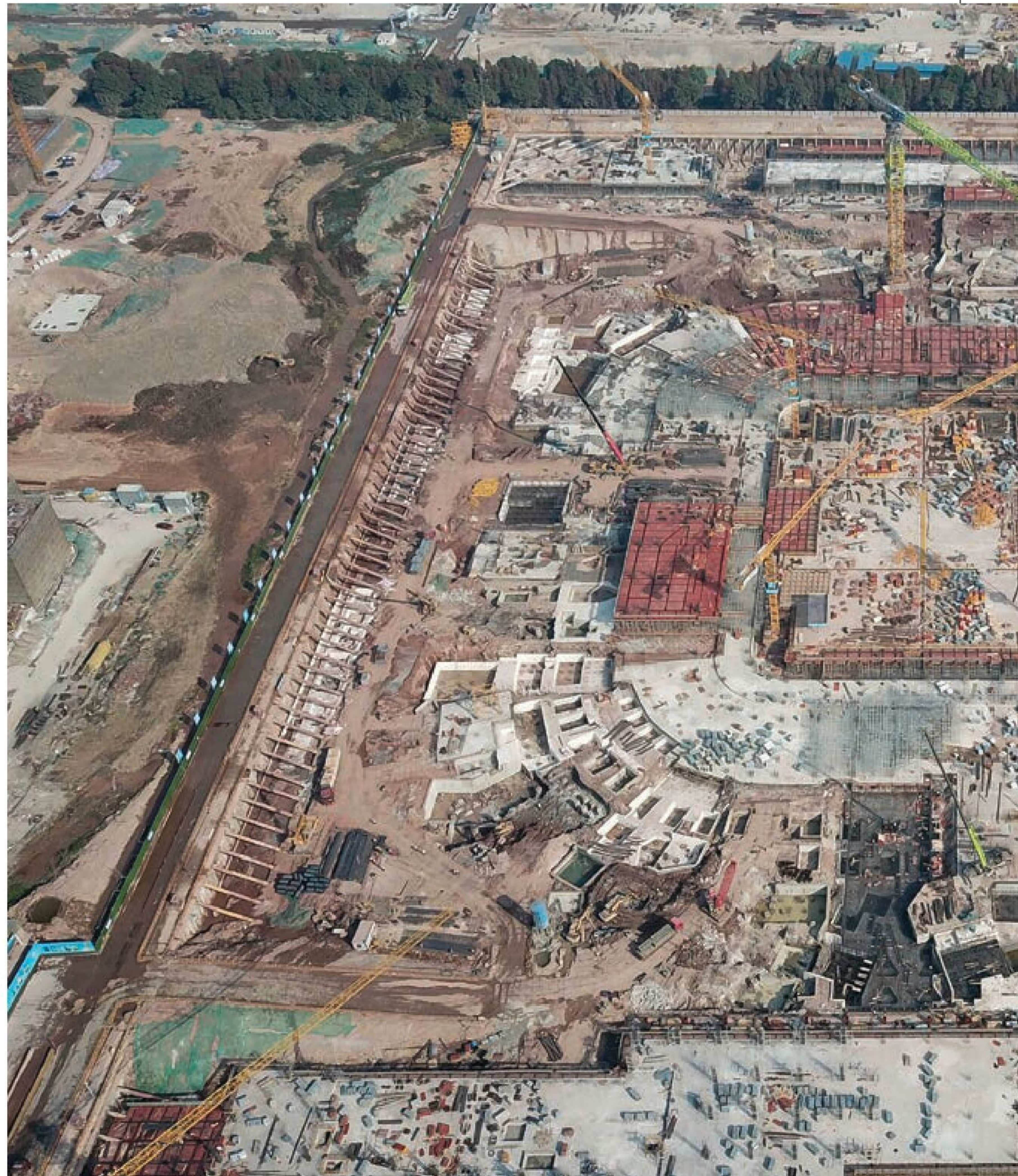
▼ Guangzhou Evergrande Football Stadium under construction in December
